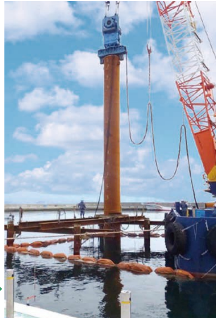
Driving through riprap seawall Steel pipe pile \phi 400 to 500\text{mm} L=16.5 to 16.7\text{m} Granite, Unconfined compression strength: q_u=80 to 130\text{MN/m}^2
