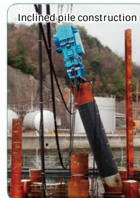
Construction is possible at up to 20°.
