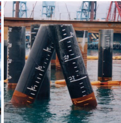
Driving through riprap seawall Steel pipe pile \phi 400 to 500\text{mm} L=16.5 to 16.7\text{m} Granite, Unconfined compression strength: q_u=80 to 130\text{MN/m}^2
