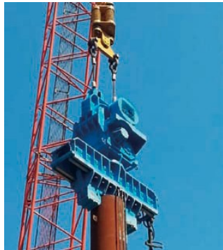
Specialized vibratory hammer "GANPILER".
