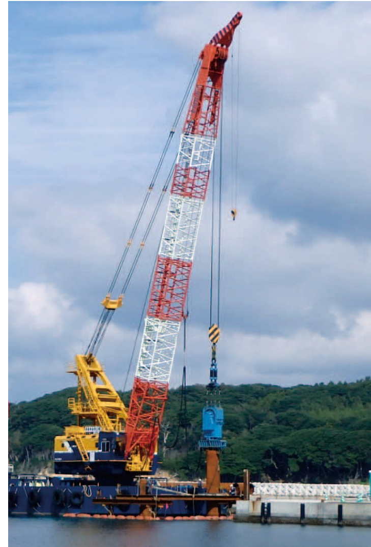
Rock Pile Driving (GANPILE) Method Research Society
